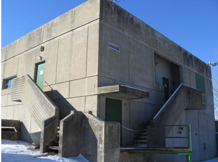
This is the water treatment facility at 1311 Adams Ferry Road in Pantown
